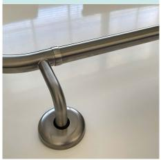
15. Ensuring rail is level, slide up flange cover and secure screws. Repeat for all fixing points.
