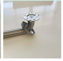
7. Ensuring rail is level, slide up flange cover and secure screws. Repeat for all fixing points.
