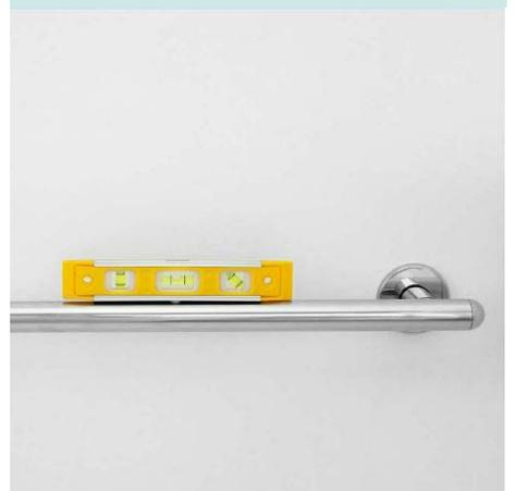
9. Position flange cover so the hole is over the screw fixing point. Secure the first screw.
