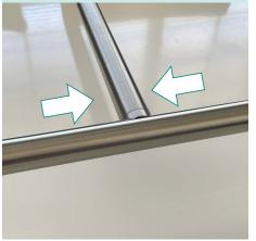
11. Ensuring rail is level, slide up flange cover and secure screws. Once complete, slide flange cover into place.
