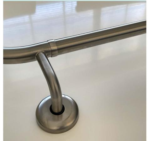
15. Ensuring rail is level, slide up flange cover and secure screws. Repeat for all fixing points.
