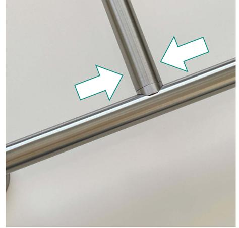
20. Ensuring rail is level, slide up flange cover and secure screws. Once complete, slide flange cover into place.
