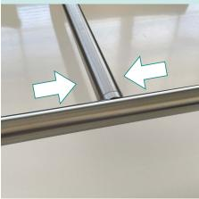
9. Ensuring rail is level, slide up flange cover and secure screws. Once complete, slide flange cover into place.
