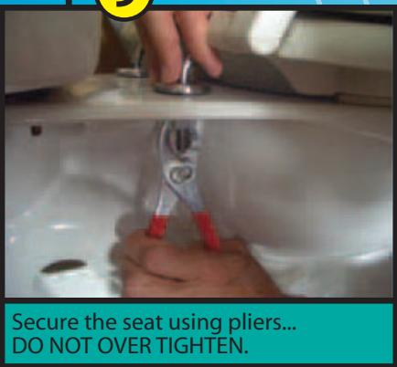
Secure the seat using pliers...
