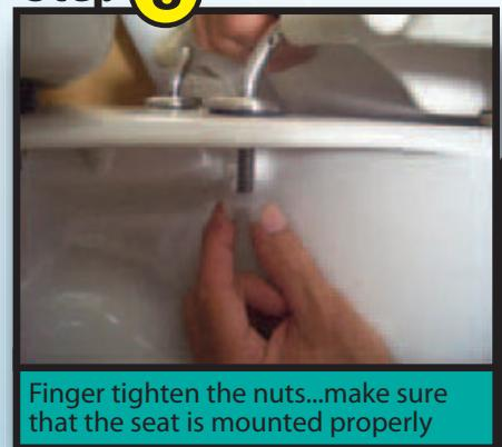
Finger tighten the nuts...make sure that the seat is mounted properly
