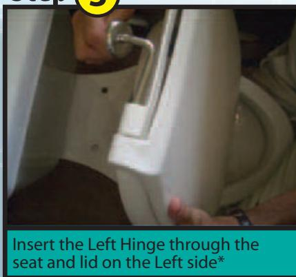
Insert the Left Hinge through the seat and lid on the Left side\*
